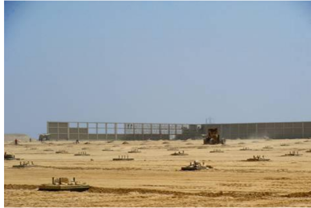
Figure 16 Construction site of parabolic trough solar field at Kuraymat (Egypt) with the foundations of the solar field
