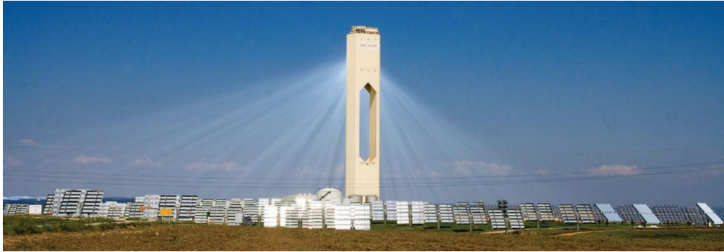
Figure 8: 11 MWe el Power Tower by Abengoa, hundreds of Heliostats concentrate the sun (up to 500 times) onto an absorber on the top of the tower
