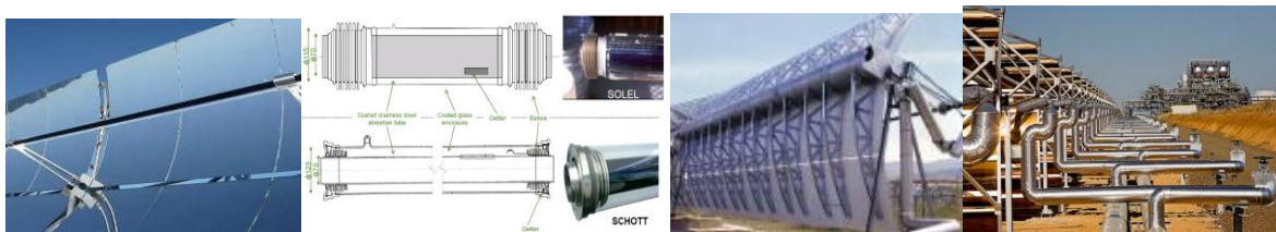
Figure 7 Mirrors, receivers, support structure, and piping for CSP plants
